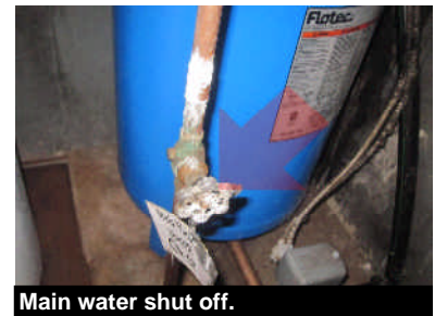
Main water shut off.
