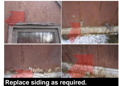
Replace siding as required.
