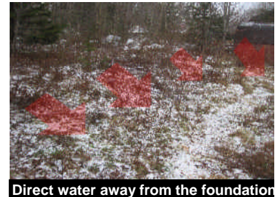
Direct water away from the foundation
