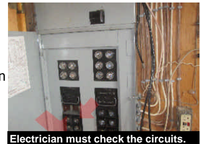
Electrician must check the circuits.
